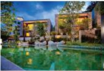
NATURAL PARK PAVILLION
